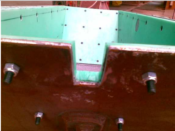
Photo 002 – End view of similar adjacent chute U034313 showing lining around cut-out
