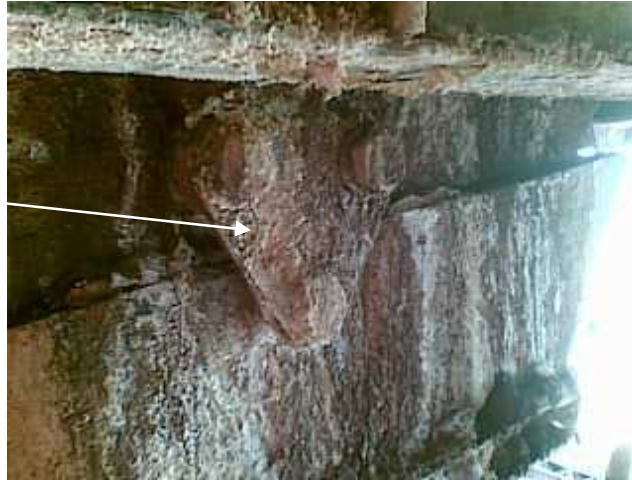
Photo 007 – Triangular pivot bracket on west side of diverter chute
