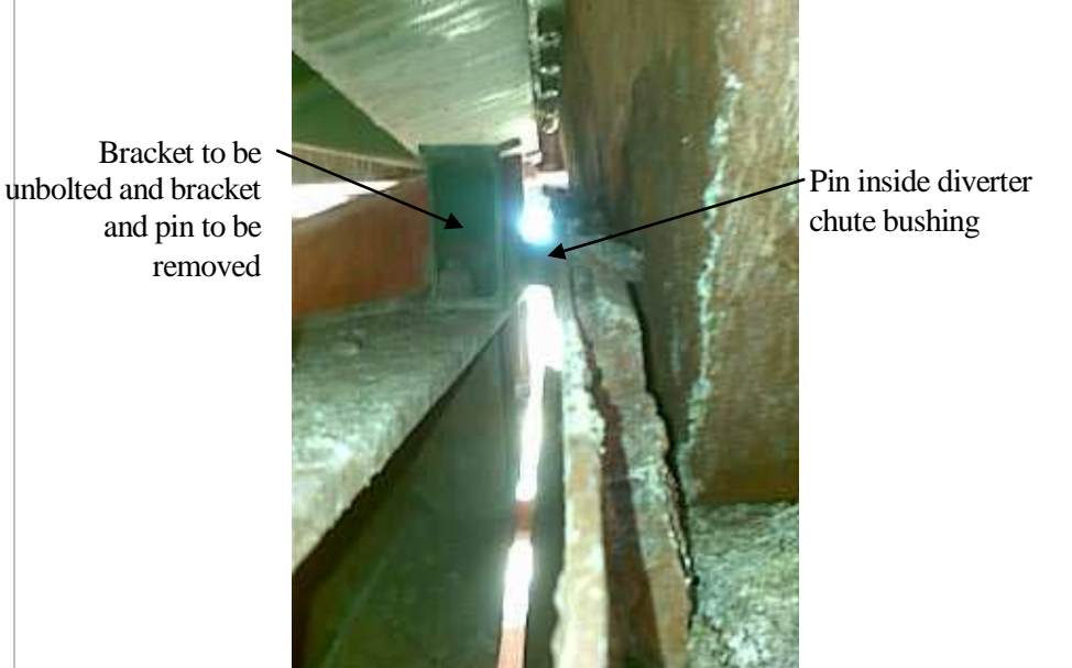
Photo 006 – Pivot bracket on east side of diverter chute
