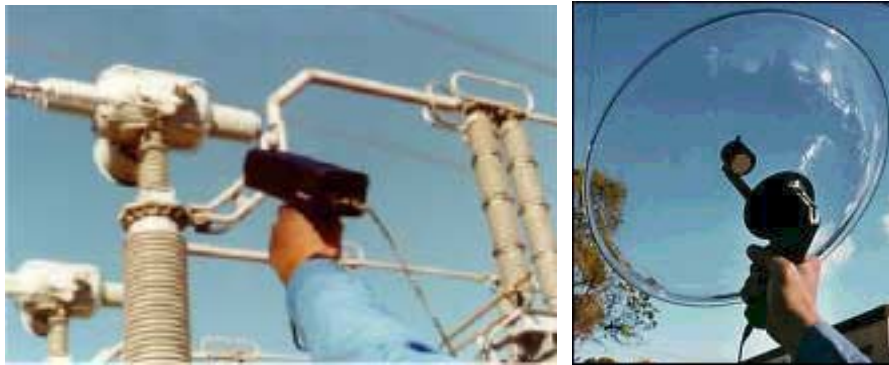
Ultrasonic Monitoring for High Voltage Tracking, Arcing and Corona Discharge
