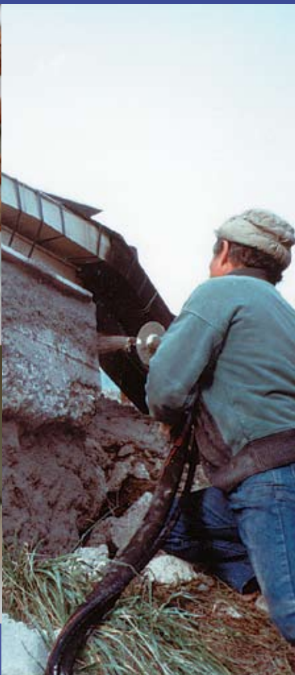
Remove spalled concrete from deteriorating structure.
