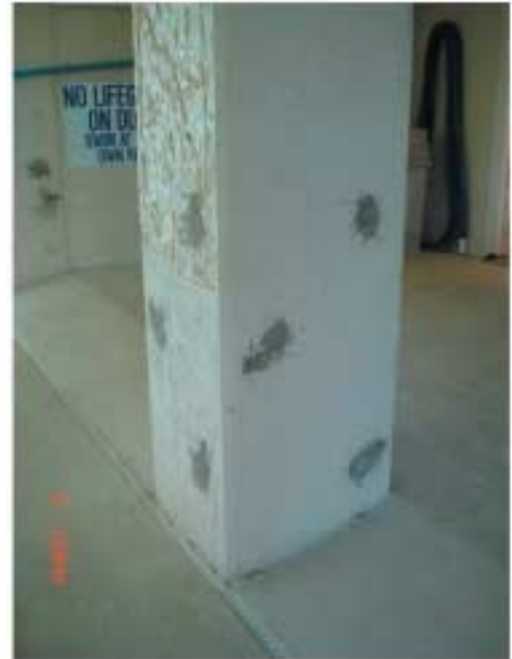
Finished Condominium Column with Galvashield CC's Installed.
